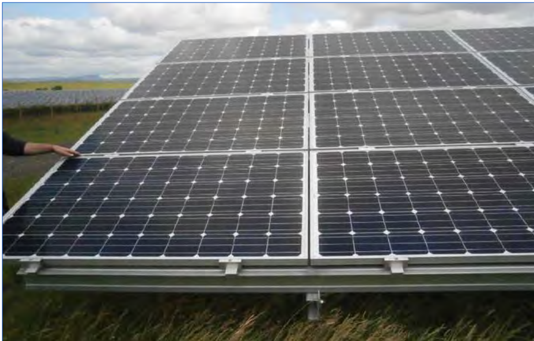
Figure 7-1 Typical Solar Panel Arrangement (showing expansion gaps)
